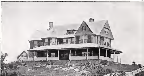
Residence of Mrs. E. K. Brazier, Kennebunkport, Me. John Calvin Stevens, Portland, Me., Architect.
